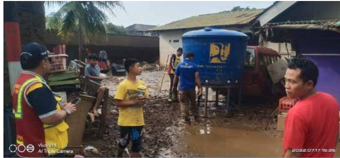
FIGURE 5. Clean Water installation in Cimacan, Tarogong Kidul District
