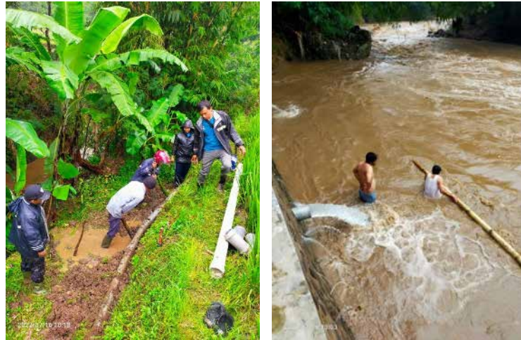
FIGURE 6. Post-disaster repair relocation of Garut City/Up Cibuntu Branch
