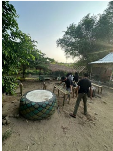
Figure 1. Bamboo Chair Installation Process
