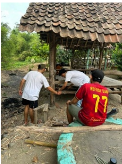
Figure 2. Water Reservoir Pole Casting
