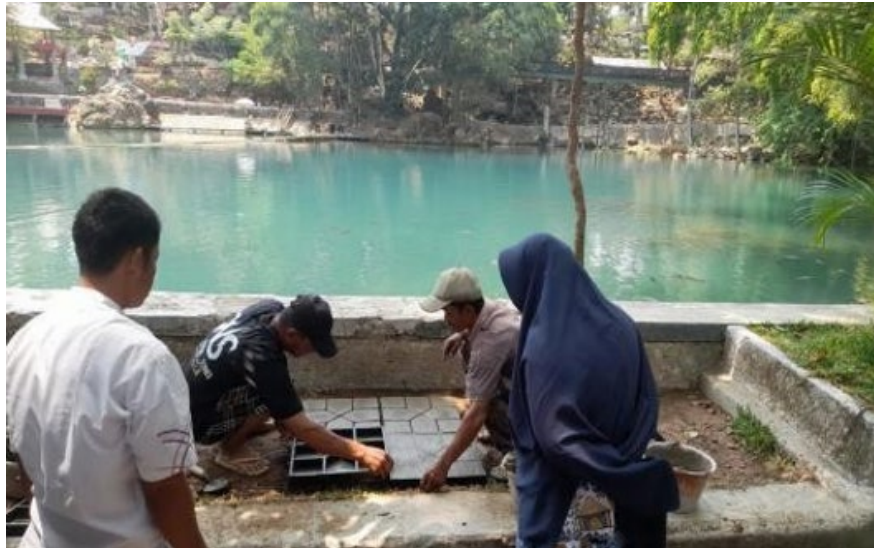
Figure 8. Making Paving Blocks
